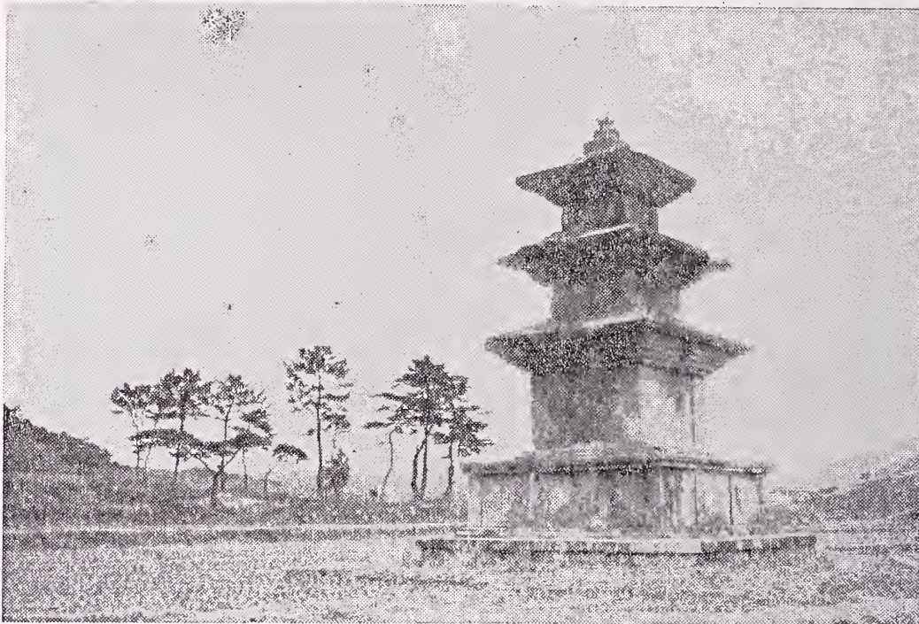
This three-story pagoda on the site of Koson-sa, near Kyongju, is National Treasure No. 38. It is one of the largest of its kind in Korea.
